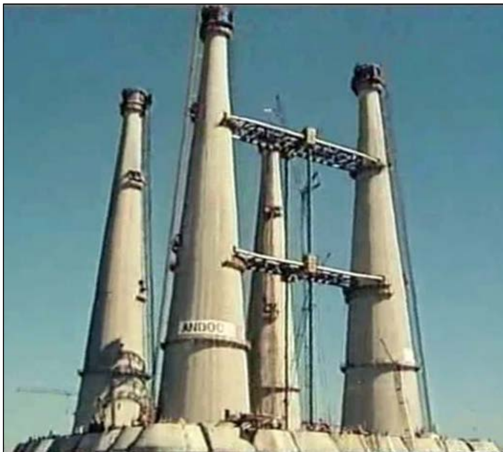
Figure 2-5: Dunlin Alpha Concrete Legs (Construction 1976)
