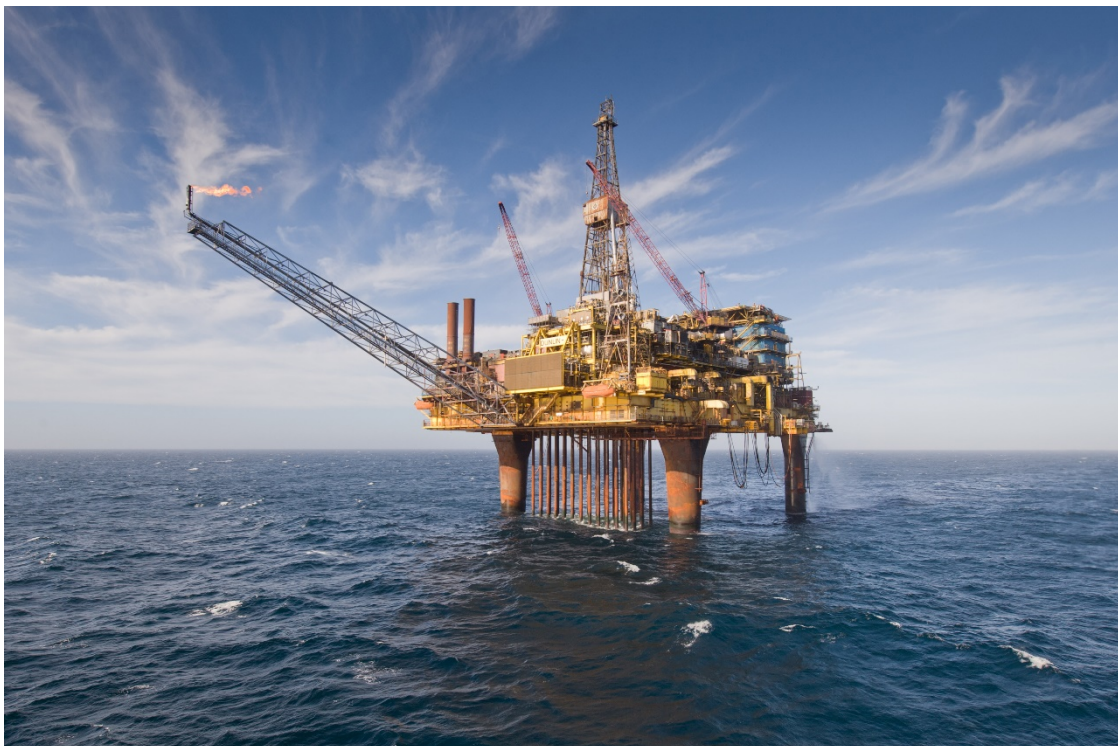
Figure 2-1: Dunlin Alpha Installation (Operational March 2012)
