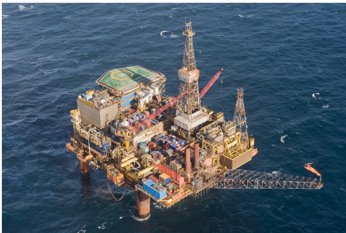
Figure 2-2: Dunlin Alpha Installation (Operational March 2012)
