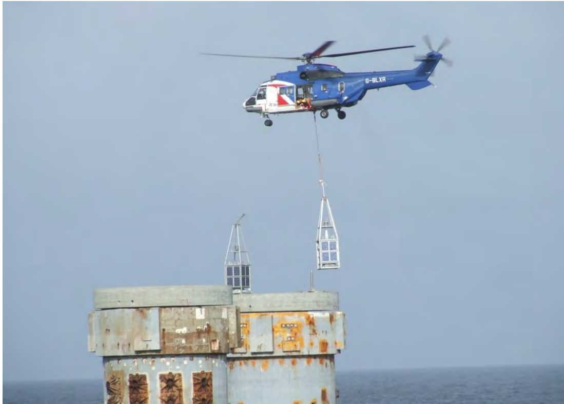
Figure 2.13 Example of a Navaid Being Installed by Helicopter
