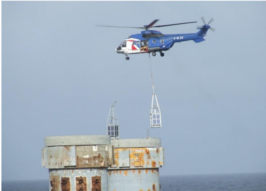
Figure 2.18 AtoN unit deployment by helicopter (Maritime Journal, 2015)
