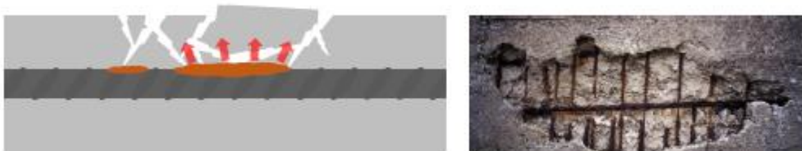
Figure 2.19 Corrosion expansion and spalling of reinforced concrete (not Dunlin Alpha)
