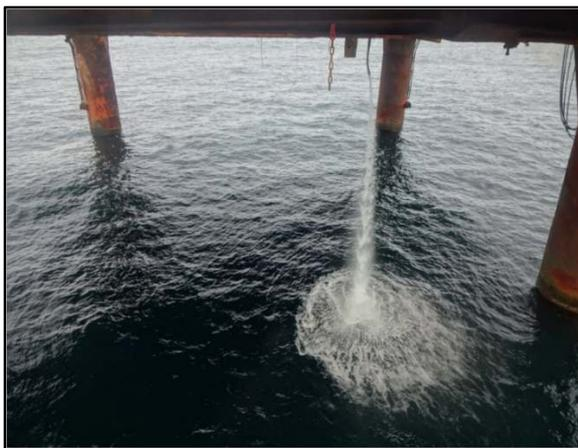
(c) Air Gap Cleared of Conductors
