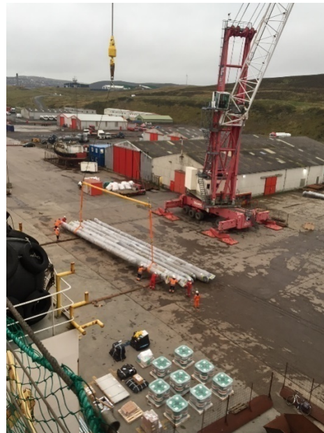
PL5 Spool Sections on Quayside
