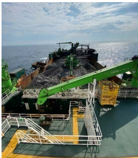
Rock Placement Operations on PL5
