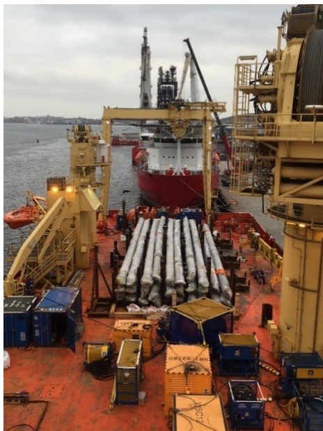
Discharge of PL5 Sections in Lerwick
