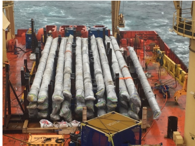
PL5 Spool Sections Recovered to CSV (Asbestos Precautions Visible)
