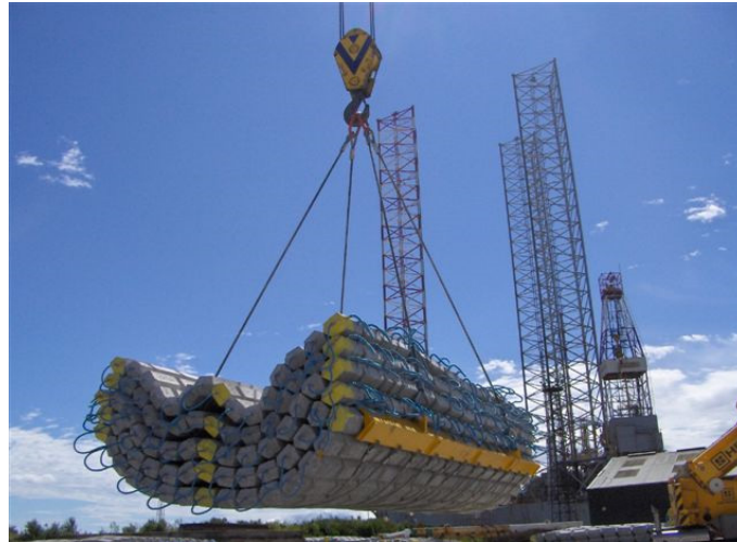
Figure 8 Illustration of multiple mattresses being lifted (system shown from Subsea Protection Systems)
