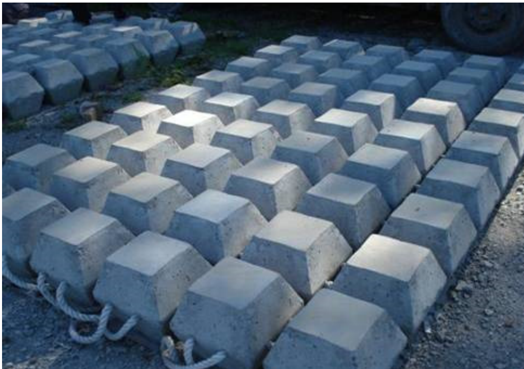
Figure 2.2 Example of a typical concrete mattress
