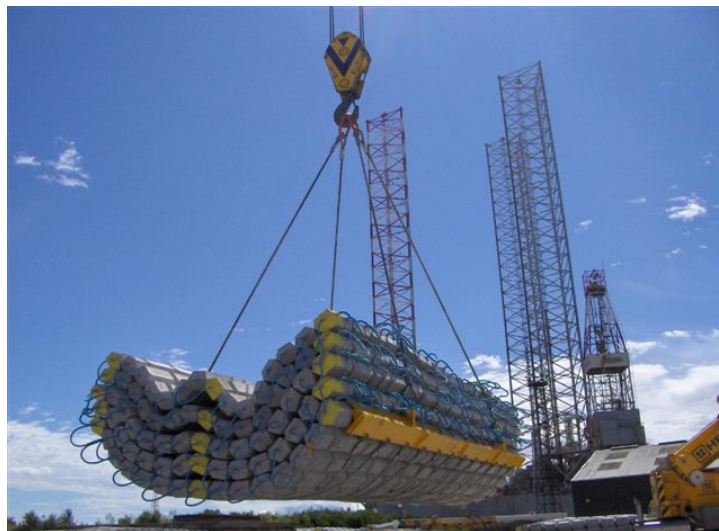
Figure 2.8 Illustration of multiple mattresses being lifted from the sea floor (system shown from Subsea Protection Systems, 2017)
