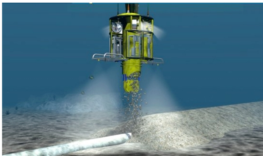
Figure 4 Illustration of a flexible fall pipe being used to deploy rock (system shown from Offshore Fleet)
