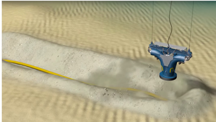
Figure 7 Illustration of a pipeline being exposed by a jet of water from a mass flow excavator (system shown from N Sea)
