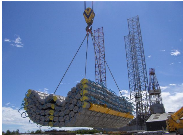
Figure 2.9 Illustration of multiple mattresses being lifted from the sea floor (system shown from Subsea Protection Systems, 2017)
