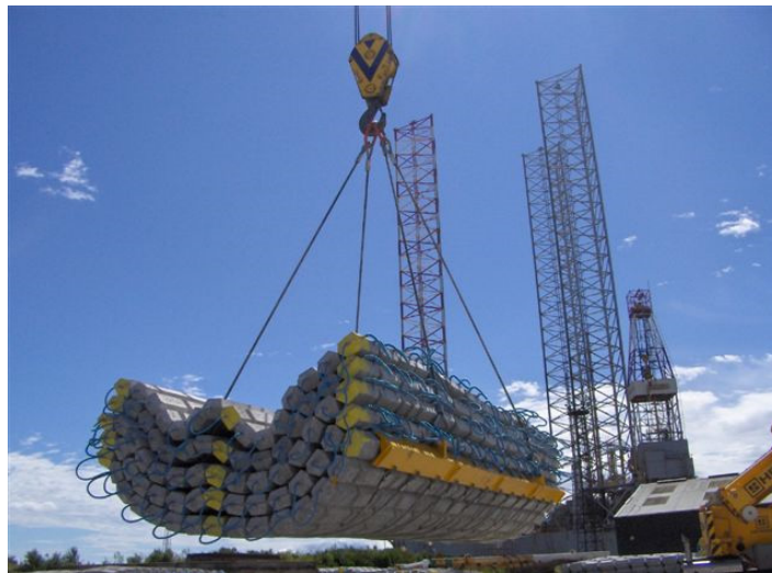
Figure 8 Illustration of multiple mattresses being lifted (system shown from Subsea Protection Systems)
