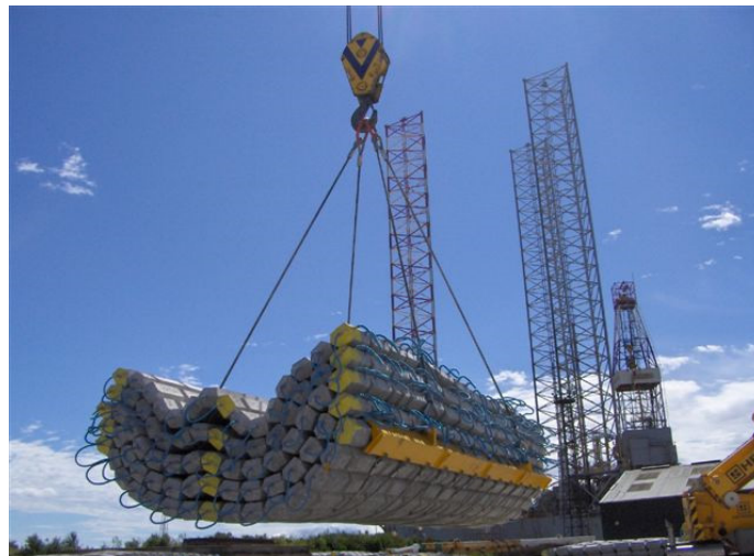
Figure 2.7 Illustration of multiple mattresses being lifted from the sea floor (system shown from Subsea Protection Systems, 2017)
