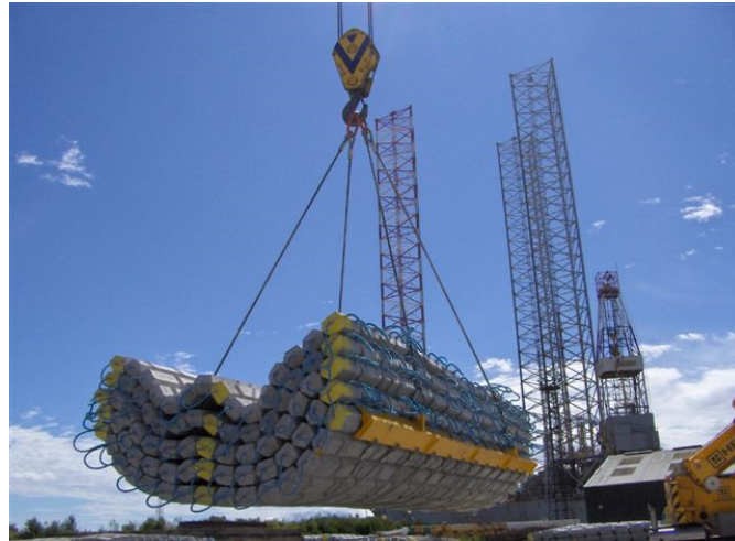
Figure 6 Illustration of multiple mattresses being lifted (system shown from Subsea Protection Systems)
