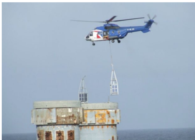
Figure 2.5 AtoN Unit Deployment by Helicopter
