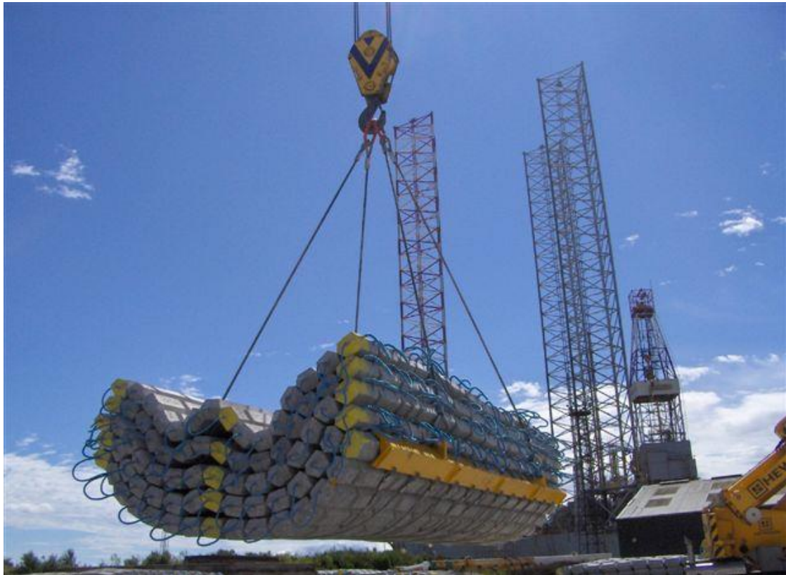
Figure iii Illustration of multiple mattresses being lifted (system shown from Subsea Protection Systems)
