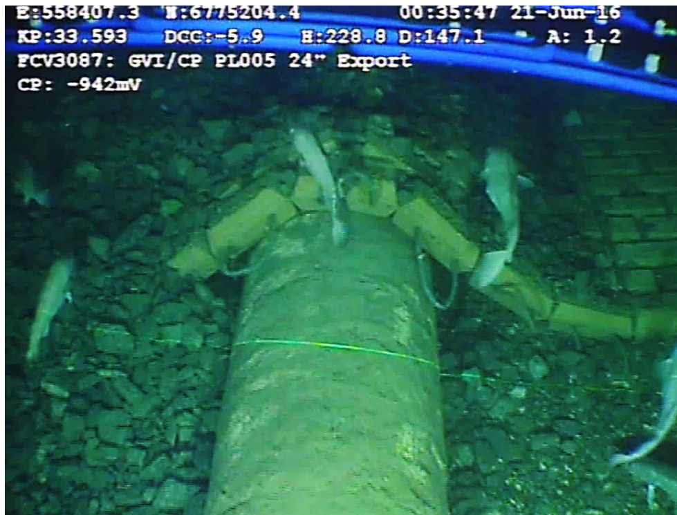
Figure 2.3 Typical mattress coverage - 2016 survey footage
